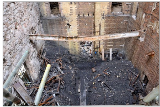
Figure 10 – Main contractor office level 2
