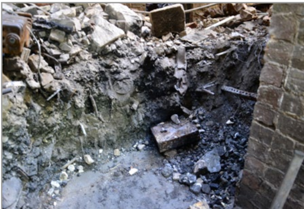
Location of FWS control panel
