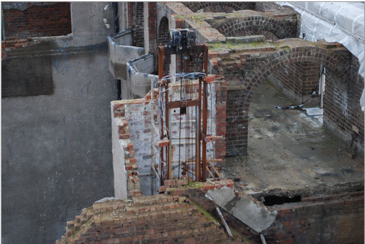
Figure 21 – Top of lift mechanism, west side
