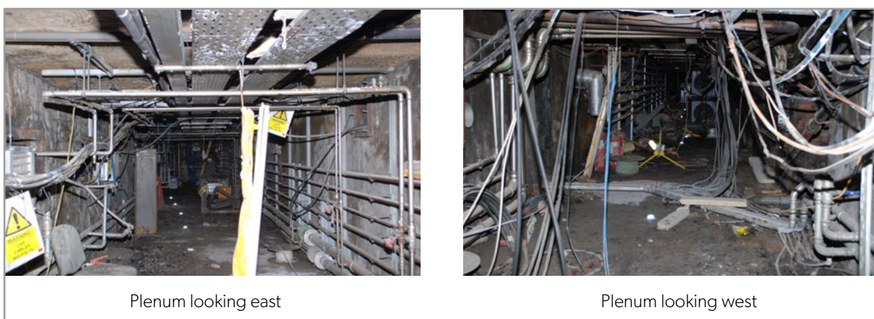
Figure 18 – Plenum below level 2
